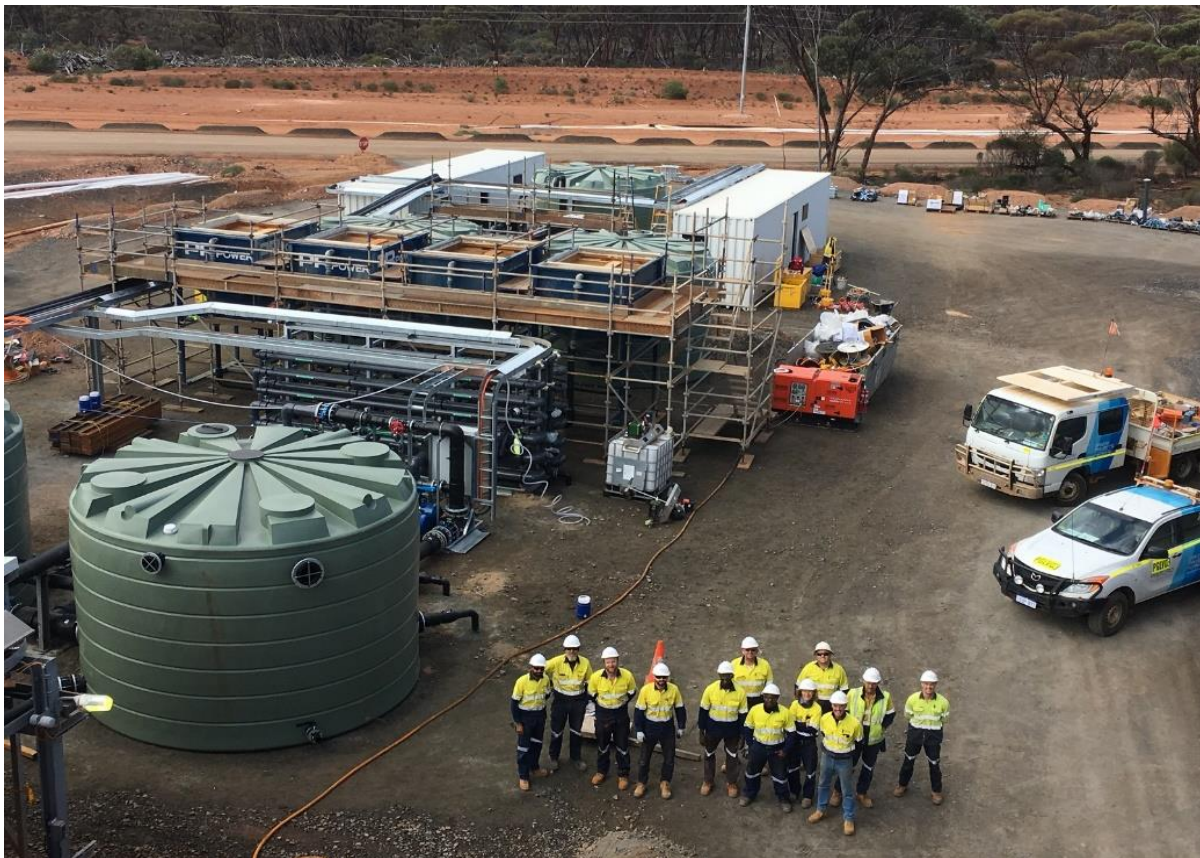
Figure 2 – Sustaining capital works at IGO’s Nova Nickel site.
