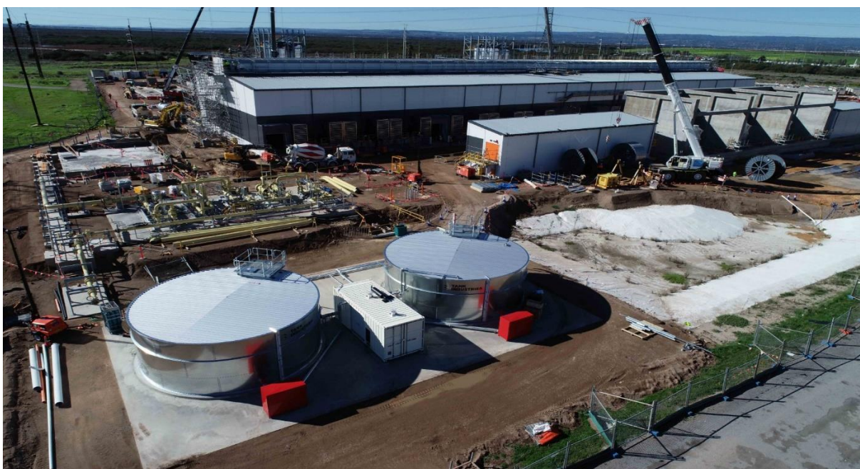
Figure 1: Progress of the Barker Inlet Power Station construction works – July 2019.
