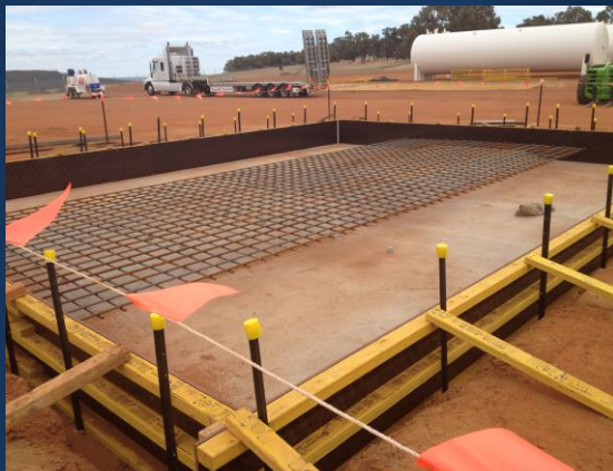
The fabricated material including pipe fittings (left) and the Export Compressor foundation slab
